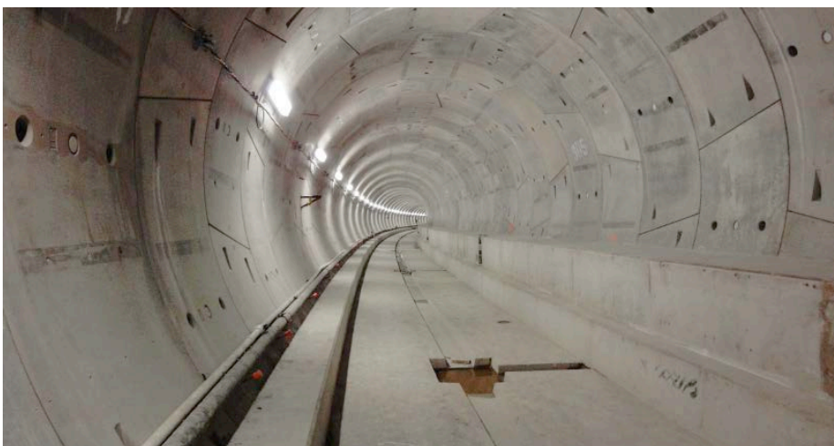
Overview of one of the completed TBM tunnels.
