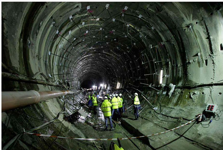
Pajares tunnel work team.
